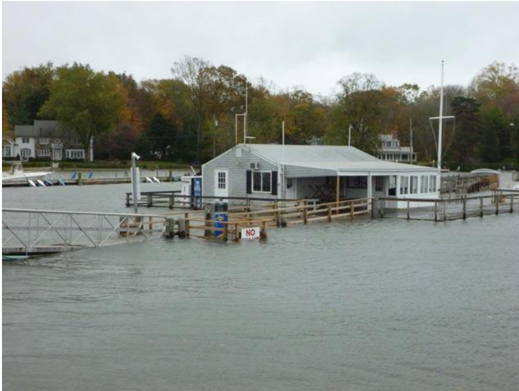
The picture shown above is of the noon tide when the wind was coming from the North. The main damage was done during the evening tide when the wind and waves were out of the South.
